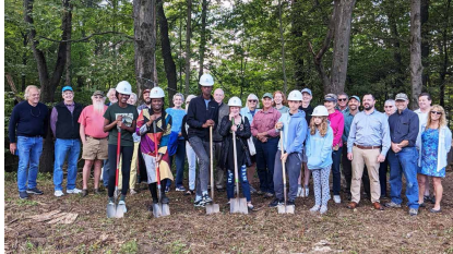
The soon-to-be homeowners are joined by volunteers, construction staff, and Habitat for Humanity folks for the ceremonial groundbreaking of a new duplex on Central Street. (Provided)
